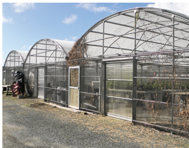
Figure 5.9 —Greenhouses are covered with transparent coverings such as plastic sheeting or hard plastic panels to maximize the amount of sunlight reaching the crop. Photo by Brian F. Daley.
